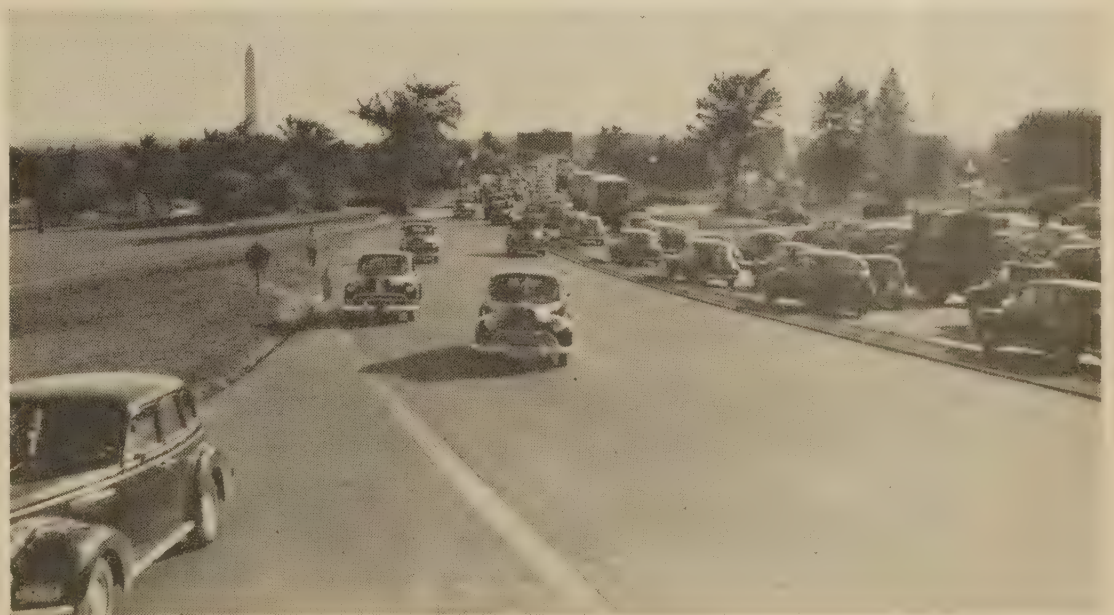
Exit turn from an expressway at a grade separation. Two lines of traffic can enter a ramp if they are in the two lanes of the expressway adjacent to the ramp, and if the drivers in the second line can be sure that all vehicles in the first line are destined for the ramp.
